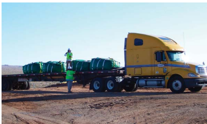
Supersacks containing radiologically contaminated material from the Highway 160 Site are being shipped on flatbed trucks to Colorado for disposal.
