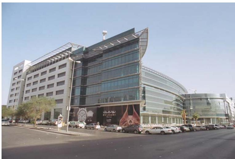
S&K Aerospace's new office is located in Riyadh, Saudi Arabia, in the Al-Aqaria Commercial Center in the Olaya District.
